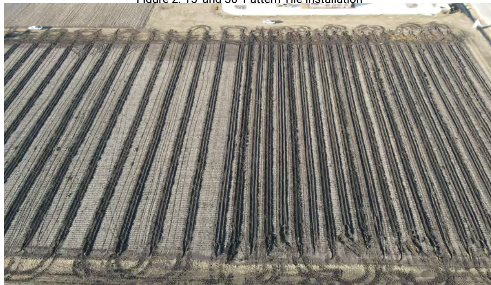
Figure 2. 15' and 30' Pattern Tile Installation
