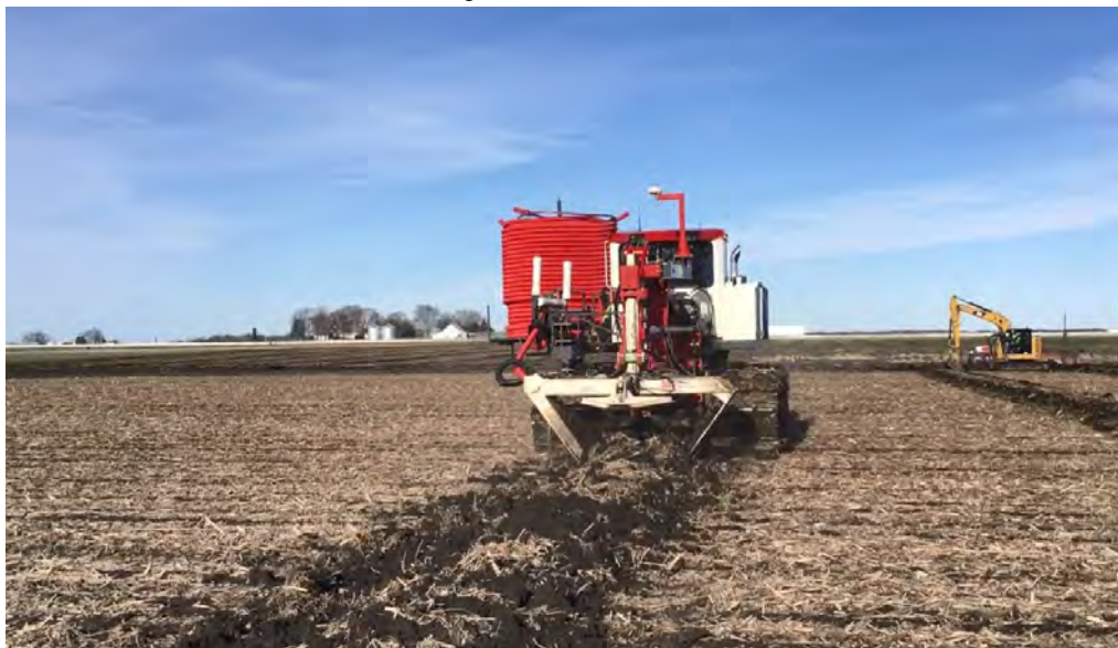
Figure 1. Tile Installation
